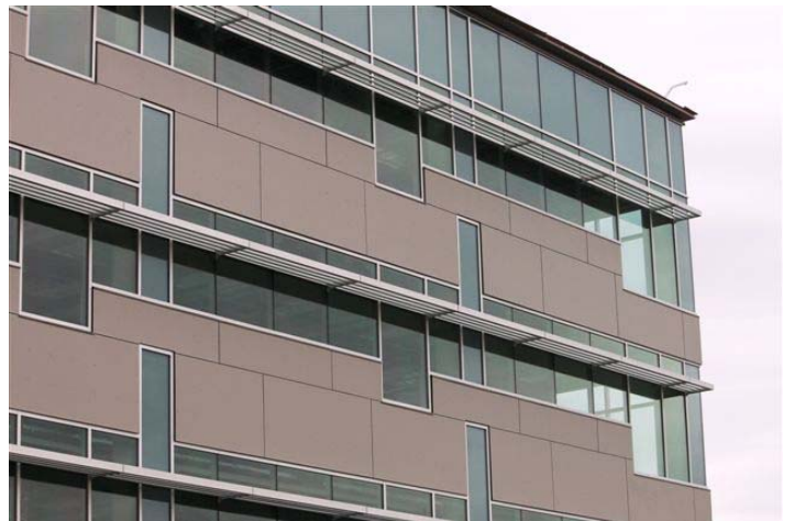
WrapShield SA Self-Adhered was installed under Trespa Meteon.
